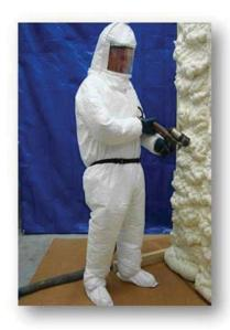
Although Personal Protective Equipment (PPE) requirements will vary depending on the type of SPF product and nature of the application, here is an example of an SPF applicator wearing proper PPE for this interior two-component high-pressure SPF installation.
